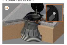
Fasten the cast iron cover at the corners with anchors bolts.
